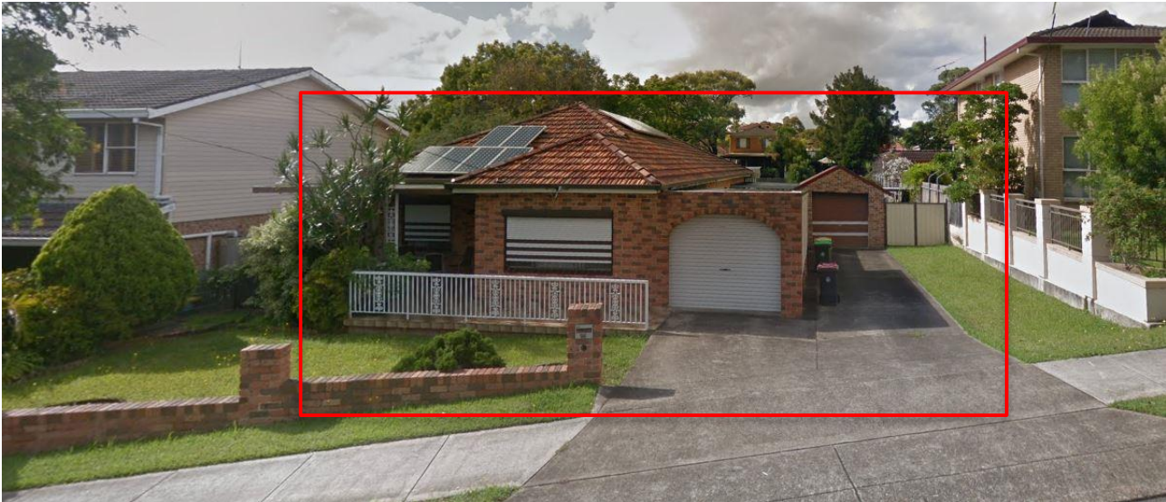
Photograph 1: View from Moorefields Road of Subject Site
